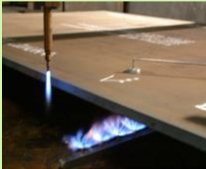
Preheating of DILLIMAX
