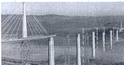
Fig. 5.5.13: Launching with pylon
