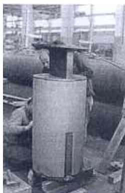
Fig. 5.5.8: Detail of the bridge bearing
