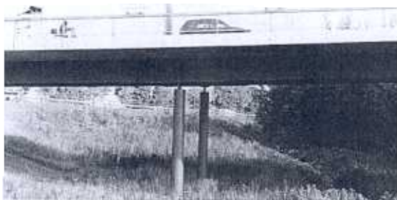
Fig. 5.5.7: Composite bridge near Ingolstadt, Germany
