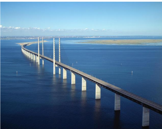
Figure 7. Higher strength thermomechanically rolled steel (S460ML) in bridge construction, Øresund Bridge, Danmark
