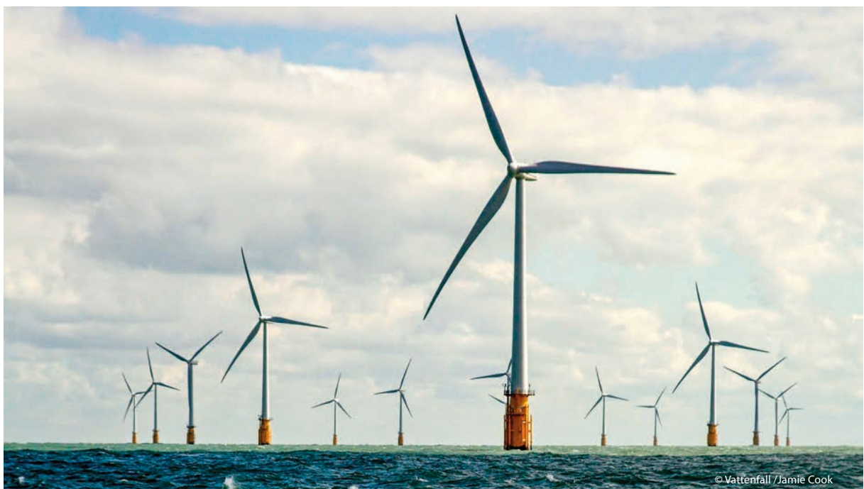
DI-MC – the reliable footing for renewable energy: the Thanet Offshore Wind Farm, constructed using thermomechanically rolled steel supplied by Dillinger
