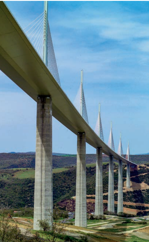
The world's longest cable-stayed bridge, France's Viaduc de Millau - was constructed using around 18,000 t of DI-MC 460 grade steel supplied by Dillinger.
