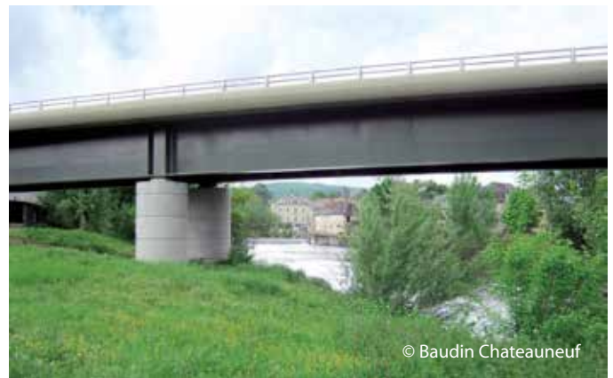
The Larche Viaduct, France, completed in 2008; 310 t of LP plates in grades S355N/NL. Plate thickness: up to 120 mm
